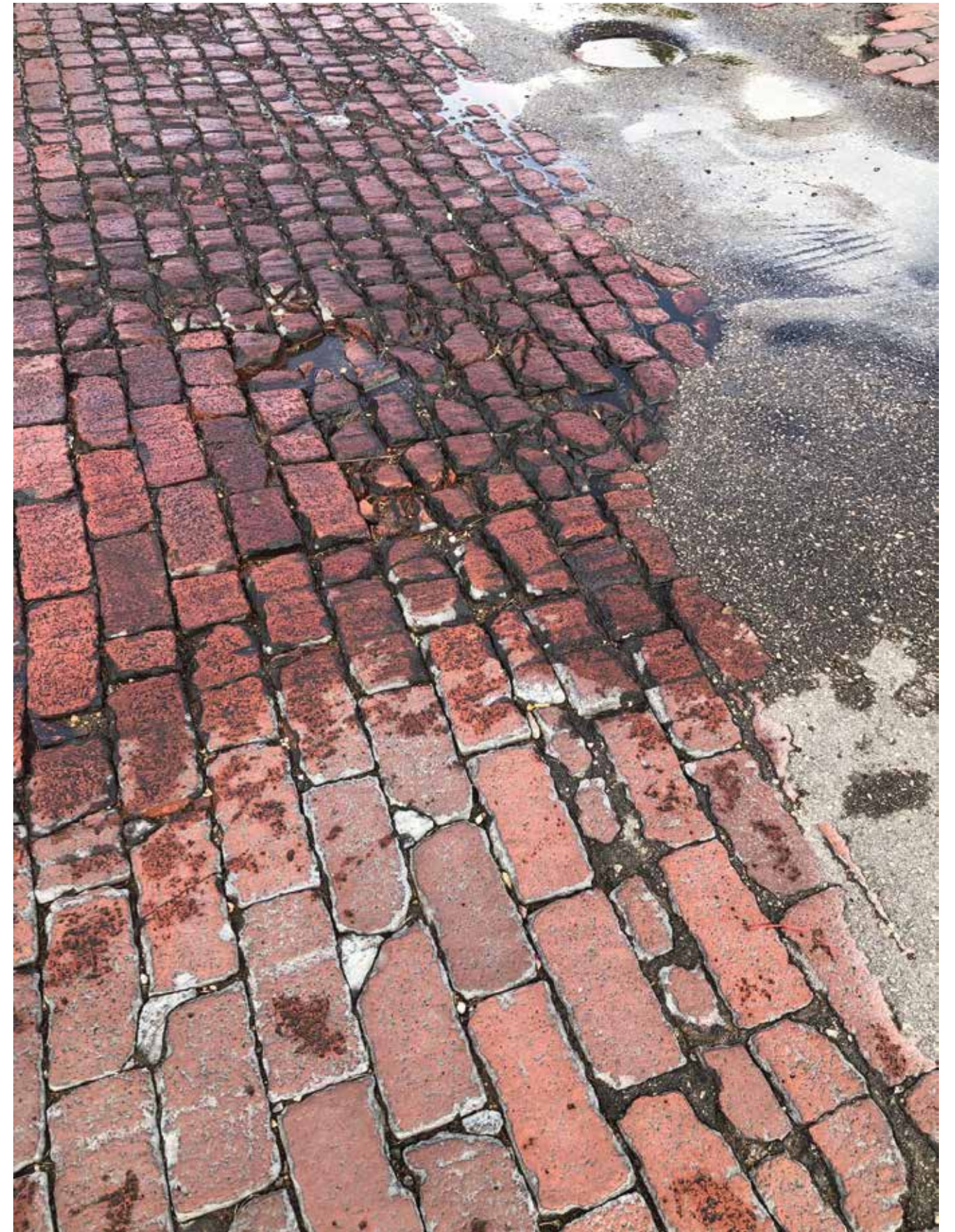
BRICK patch work
