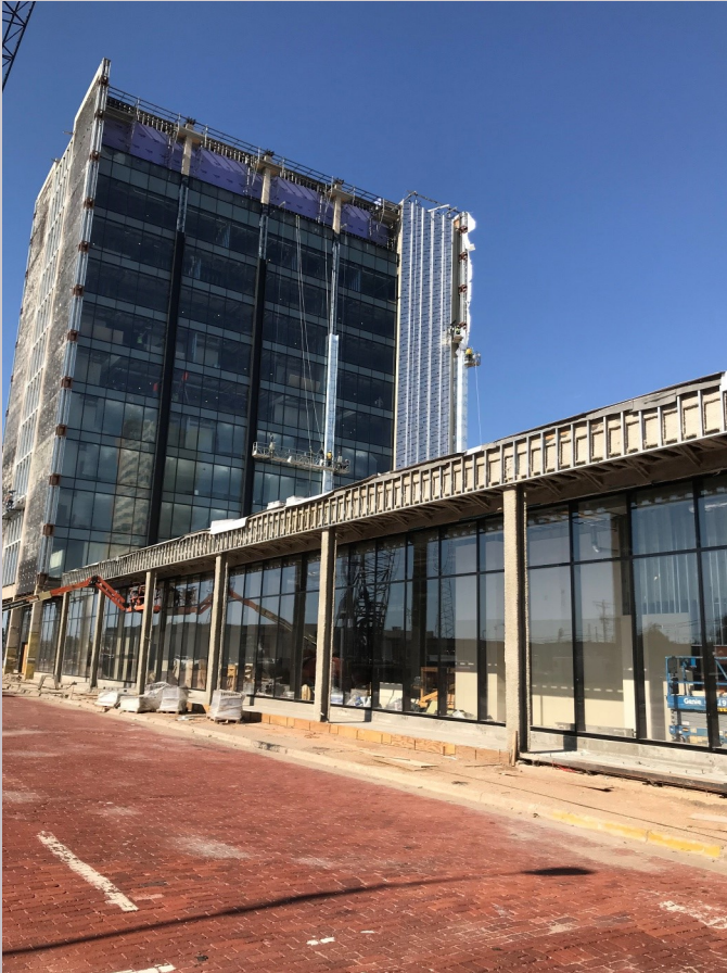
Metal panel column covers on North Tower in progress, Insulation for terracotta panels being installed.
