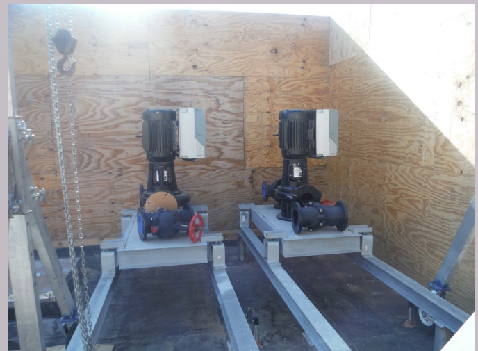
Chilled water pumps placed on low roof of Tower
