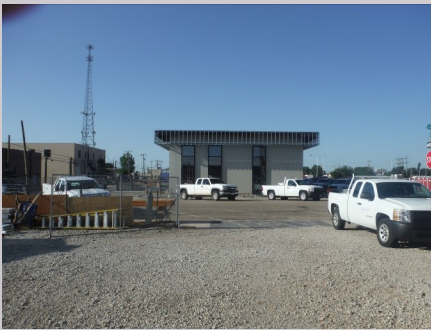
Exterior fluid applied waterproofing complete
