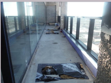
Exterior maintenance/window washing davits set into 11th floor balconies
