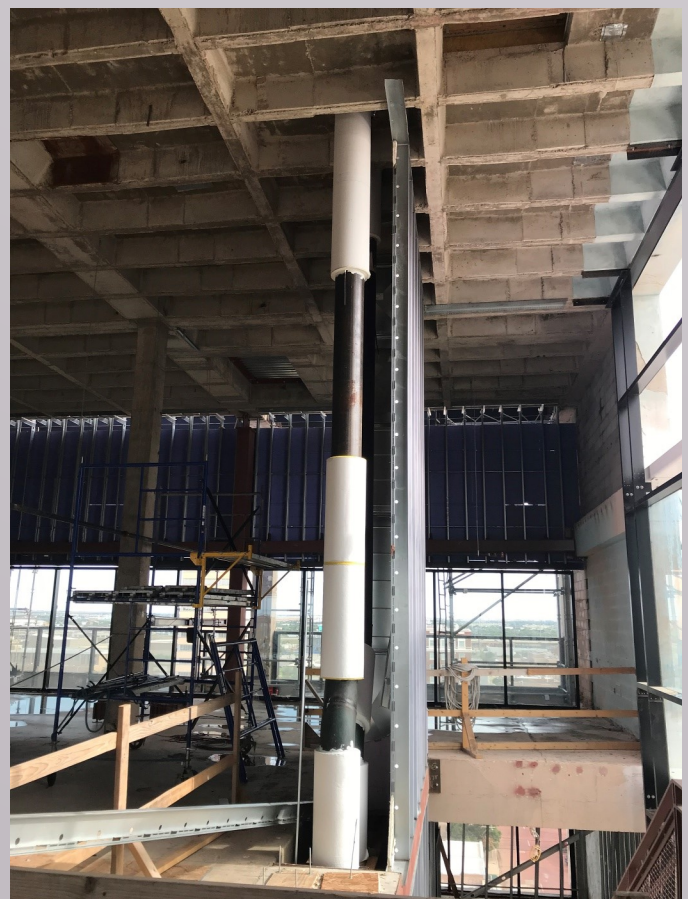
Chilled water lines extend through high roof of 11th floor Insulation in progress
