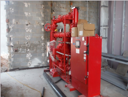
Fire pump set at 1st floor
