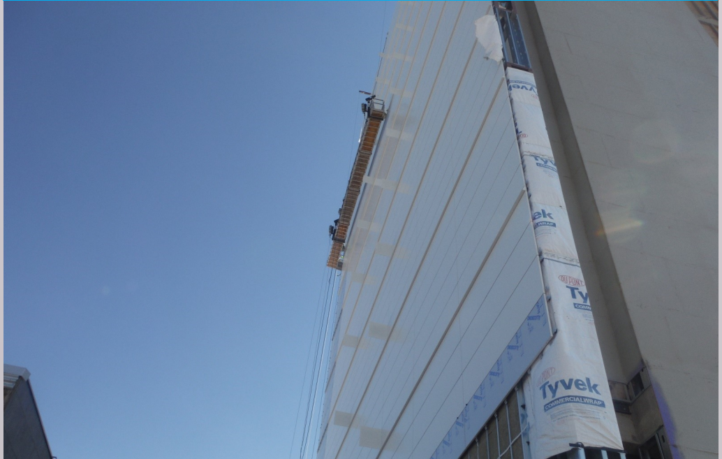
West facade metal panels in progress
