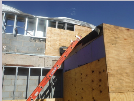
Passenger elevator penthouse & machine room at low roof
