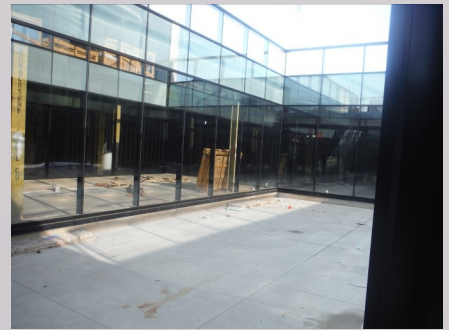
View of basement courtyard
