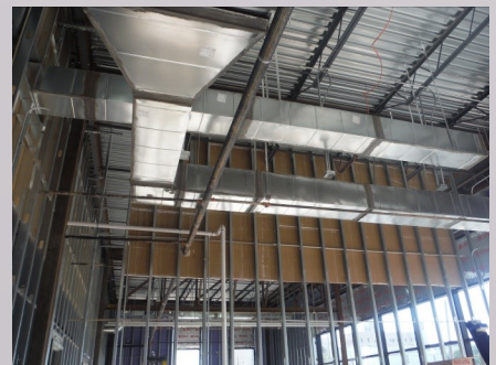
HVAC ductwork at first floor
