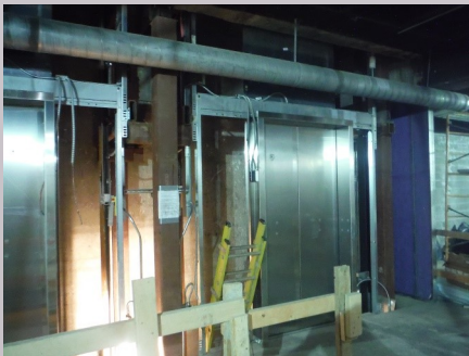
Basement elevator door panels & jambs installed
