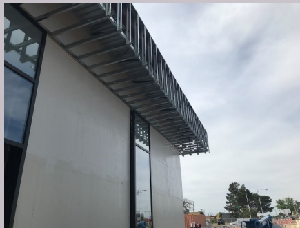
Framing for soffit and fascia complete
