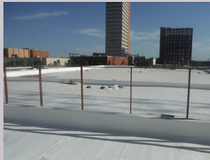
Roofing in progress
