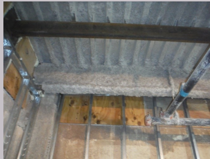
Steel fireproofing below sidewalk
