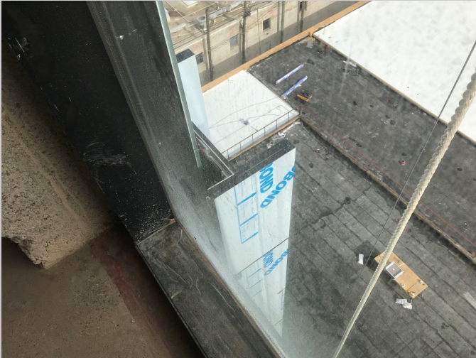
Top view of metal panel column covers at existing concrete structure
