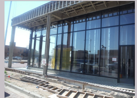
Glass installed at North facade
