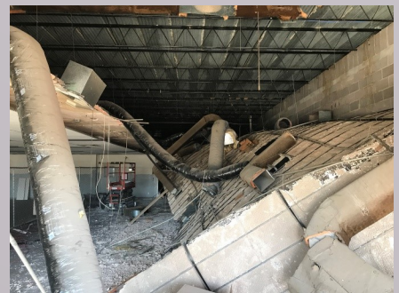
Demolition of existing interior plaster & lay-in ceilings in progress
