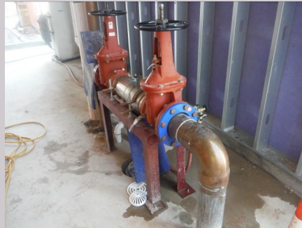
Domestic water double check valve assembly
