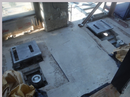
Davits are connected to structural steel located below balconies
