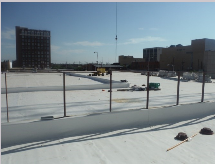
Handrail supports installed at outdoor roof terrace
