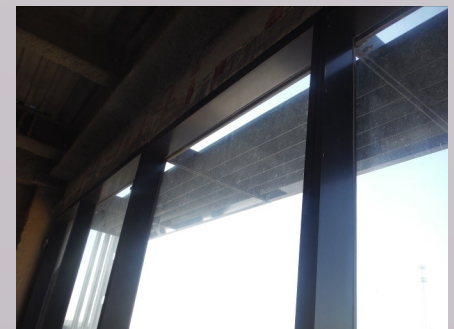
South façade passive solar shades installed on all floors
