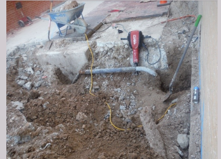
Demolition & removal of abandoned lines in progress
