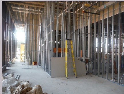
Framing continues at first floor
