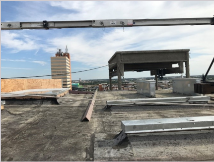
Service elevator penthouse at high roof
