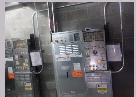
Elevator control panels at low roof mechanical room
