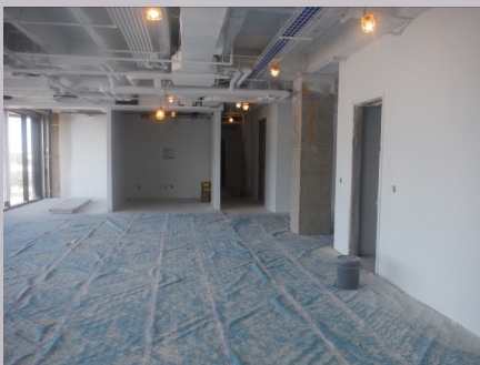
Gypsum drywall tape, bed, texture & paint begins on lower floors
