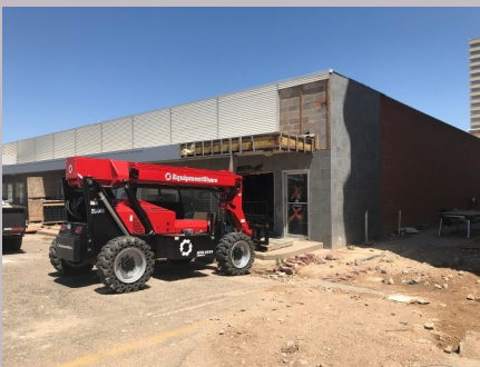
Demo begins at the corner of adjacent building for generator/transformer yard
