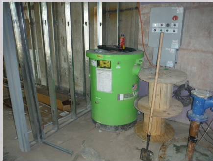
Basement elevator sump
