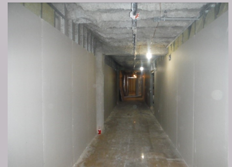
Basement gypsum drywall in progress
