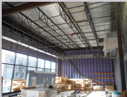
UCSC first floor progress
