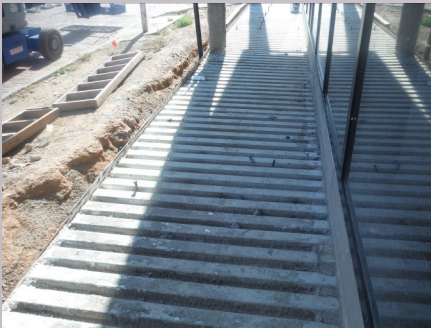
Preparing for concrete placement of sidewalk at North end
