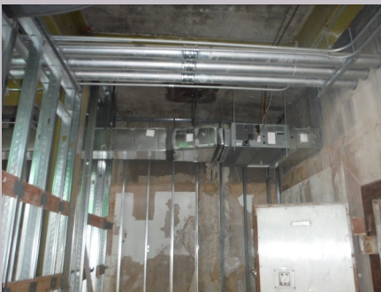
HVAC, electrical & framing work in basement
