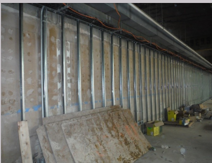
Fur out framing at perimeter basement walls
