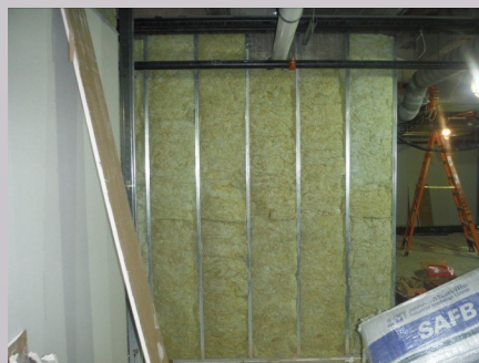
Insulation in basement walls continues
