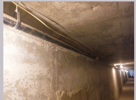
Tunnel fire sprinkler protection in progress
