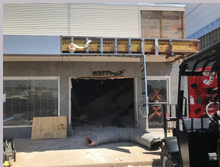
Demolition of exterior storefront
