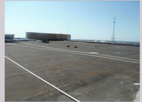
Base plies of high roof complete
