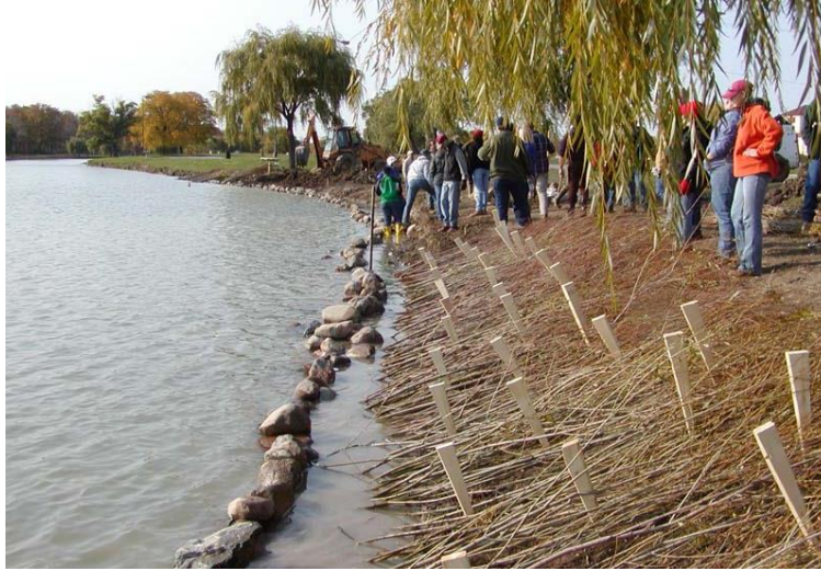
Brush mattress erosion control
