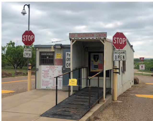
Sam Wahl Recreation Area Permit Office Source: Half Associates
