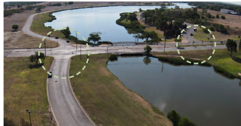
The intersection of Canyon Lakes Dr. and M.L.K. Jr. Blvd. at Dunbar Lake depicts the typical crossing conditions at Canyon Lakes parks. Existing crossings do not have signage, crosswalk markings, signals, or pedestrian medians, all while vehicles traverse a five lane roadway at 40 miles per hour. Source: Half Associates
