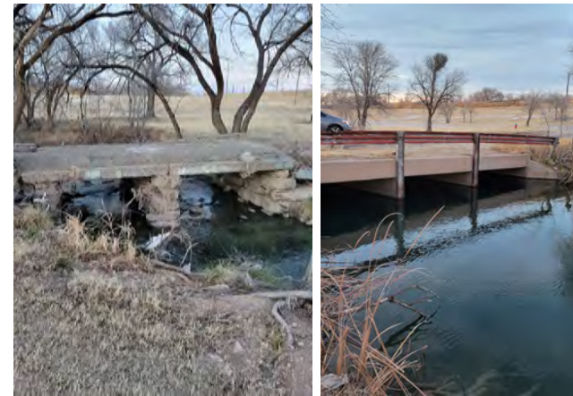
Existing bridges at the Canyon Lakes such as golf cart bridges (left) and low water / low bridge vehicular crossings (right) will need to be removed or designed to accommodate blueway users. Source: Half Associates
