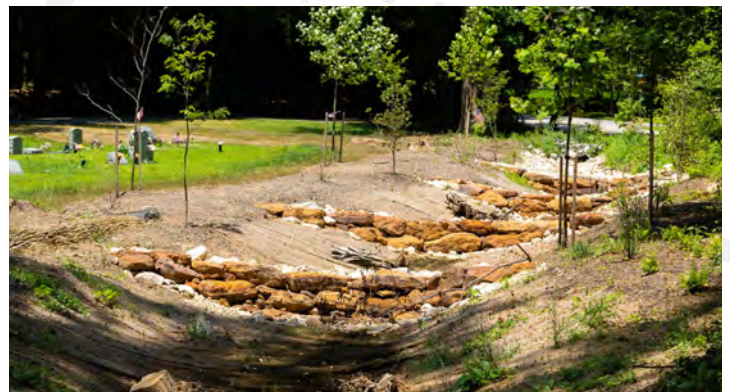
A church along the Whitehall creek in the Chesapeake Bay area created a series of step pools to reduce flood damage and stream bank erosion.
