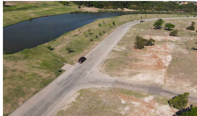
A typical view of Canyon Lakes Drive and Cesar E. Chavez Dr. at Mae Simmons Park depicting a lack of sidewalks, bicycle lane markings, signage, and pedestrian facilities. Source: Half Associates
