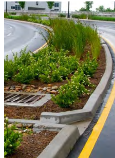
Roadway bioretention area Source: Clean Water Nashville
