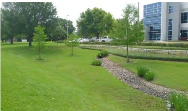
Micro-detention area with trees and other plantings Source: Construction EcoServices
