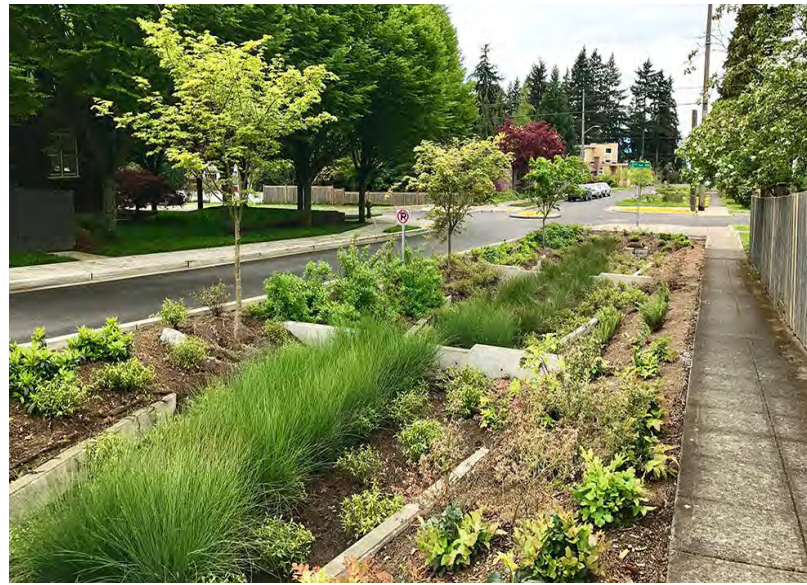
Vegetated swale along a residential street in Houston, Texas. Source: Houston Builders' Association
