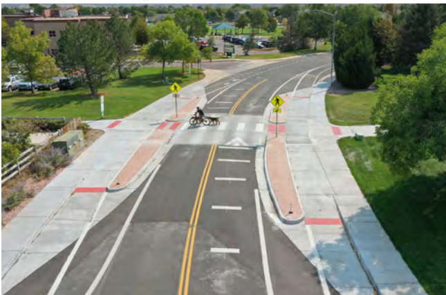
A trail crossing including a road diet, on street bicycle lanes, curb bump-outs, an elevated crosswalk table, signage, and striping.
