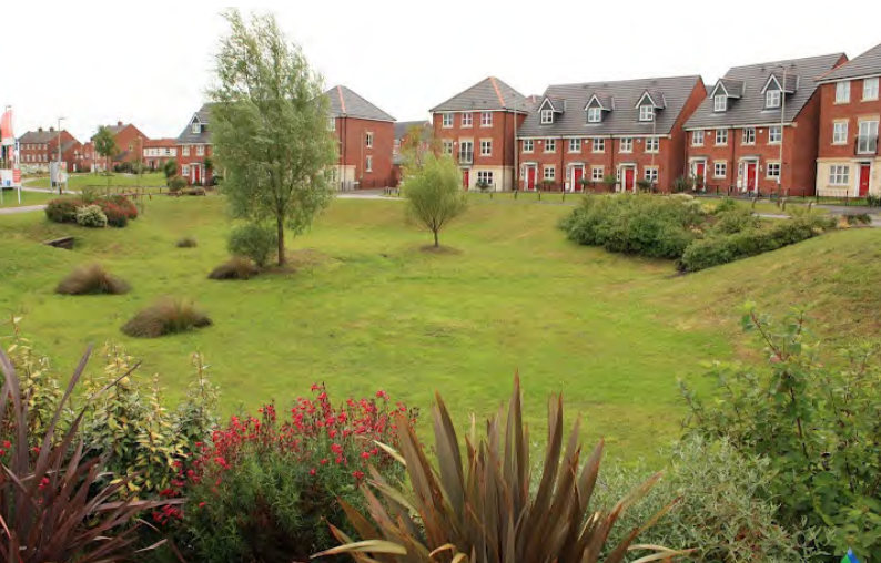
Landscaped detention ponds add visual appeal without the need for irrigation. Source: susdrain.org
