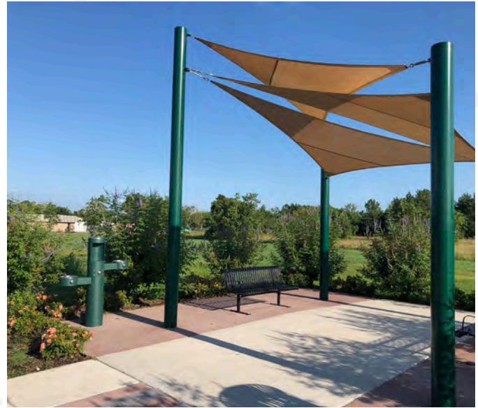
A minor trailhead along Mary's Creek Trail in Pearland, Texas, features two benches, a water fountain, waste receptacles, and a small vinyl shade structure
