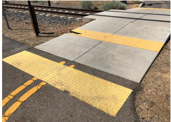
Pedestrian concrete platform crossing a rail line Source: Half Associates
