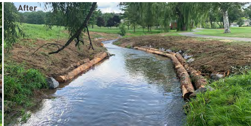
Slab Cabin Run is a stream used by migrating trout that was dredged due to narrow and shallow conditions due to erosion caused by a lack of vegetative buffers.
