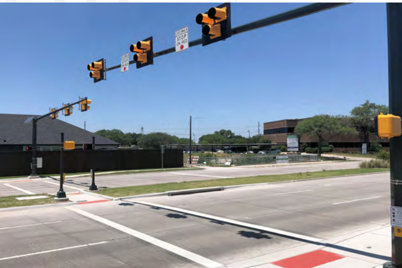
Dedicated pedestrian and cyclist crossing with flashing beacons requiring drivers to stop in either direction when a non-motist is present Source: The Colony Texas
