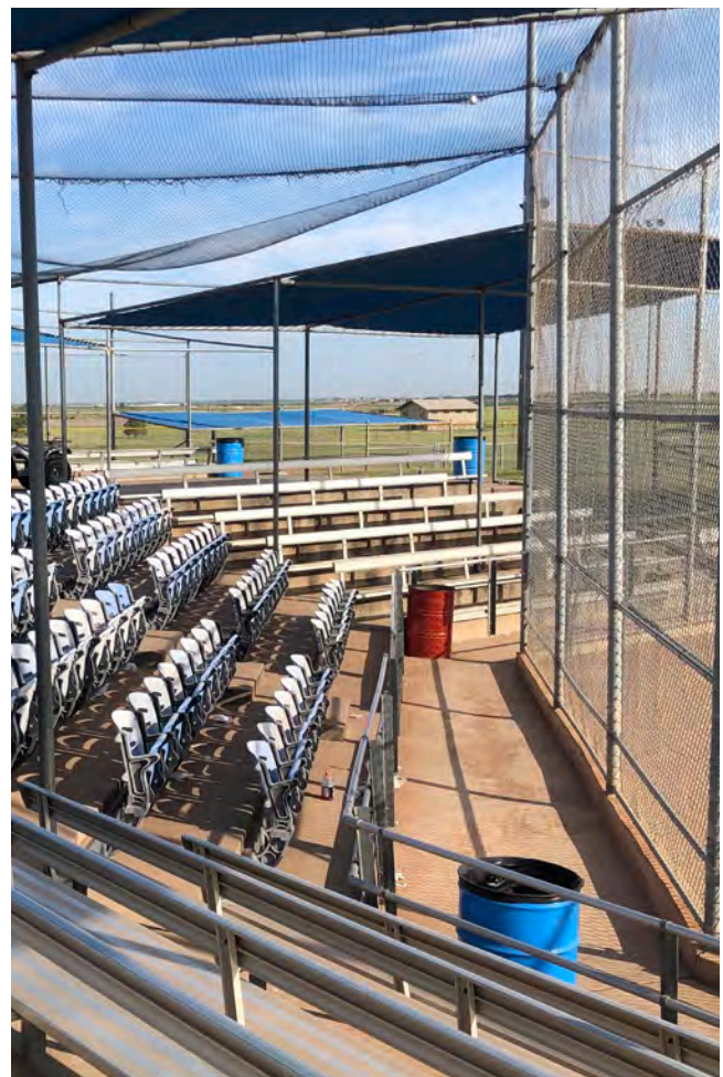
Covered Bleacher Seating at Berl Huffman Sports Complex Source: LUCK Design Team
