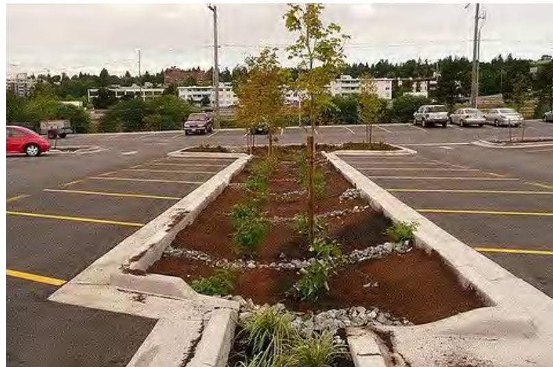
Parking lot bioretention area featuring trees and other small plants to collect rain water. Source: California Stormwater Quality Association
