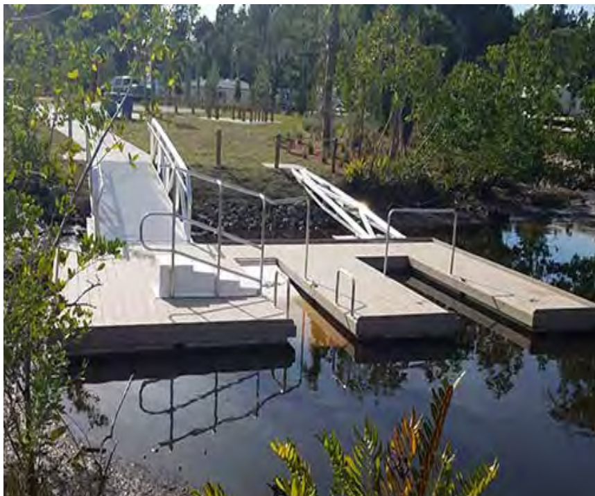
Canoe launch floating dock Source: Kay-aKcess
