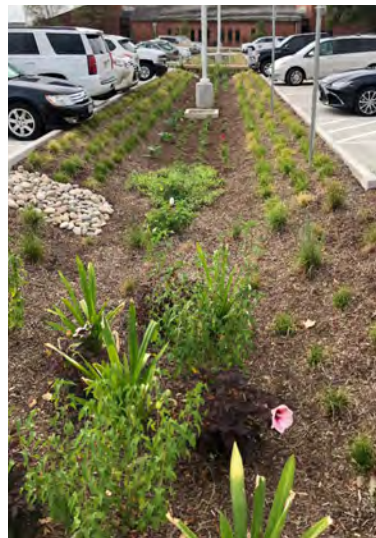
Parking lot bioretention area, Dallas, Texas Source: Texas A&M AgriLife Extension
