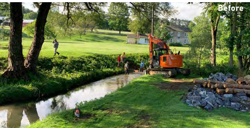
Slab Cabin Run is a stream used by migrating trout that was dredged due to narrow and shallow conditions due to erosion caused by a lack of vegetative buffers.
