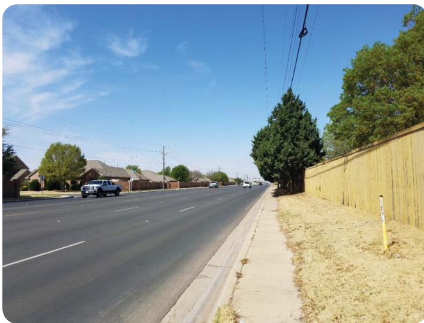
Thoroughfares provide ample space for motor vehicles but can be a barrier for walking between neighborhoods
