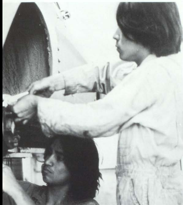
Fixing a wheel bearing takes patience and cooperation; Noey Gallivias and Joe Hernandez found this out in auto tech.
