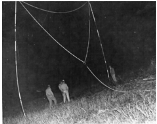
Poles with tow rope attached being set up for a night “snatch”
